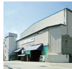
KAWAGUCHI MATERIAL CENTER
